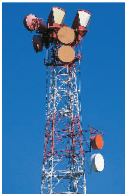
Figure 9 Towers such as the one shown here are used to send and receive microwaves.
